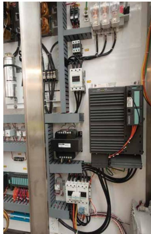
keep each pool's water moving at 30,000 gallons per minute. With its onboard CPU, the ET 200S distributed I/O nodes can offload computing tasks from the S7-300 master controller and permit much faster responses to time-critical signals.
